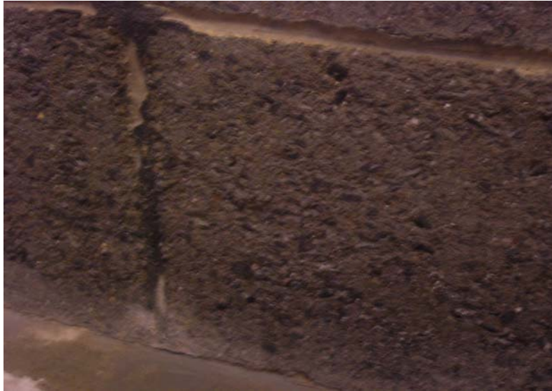
Figure 1 – Deterioration of Block Wall.
