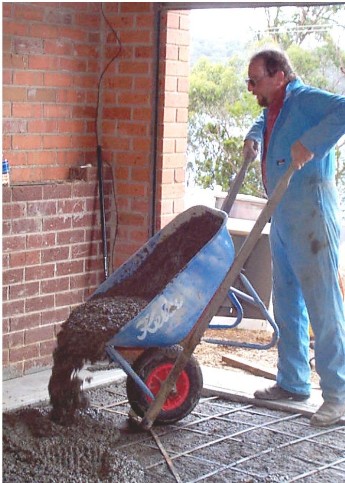
Figure 1 – Barrowing in a Low Slump Tec-Cement Concrete. Tech Tendons Laid in a Rectangular Pattern Over a First Layer Prior to Finishing with a
