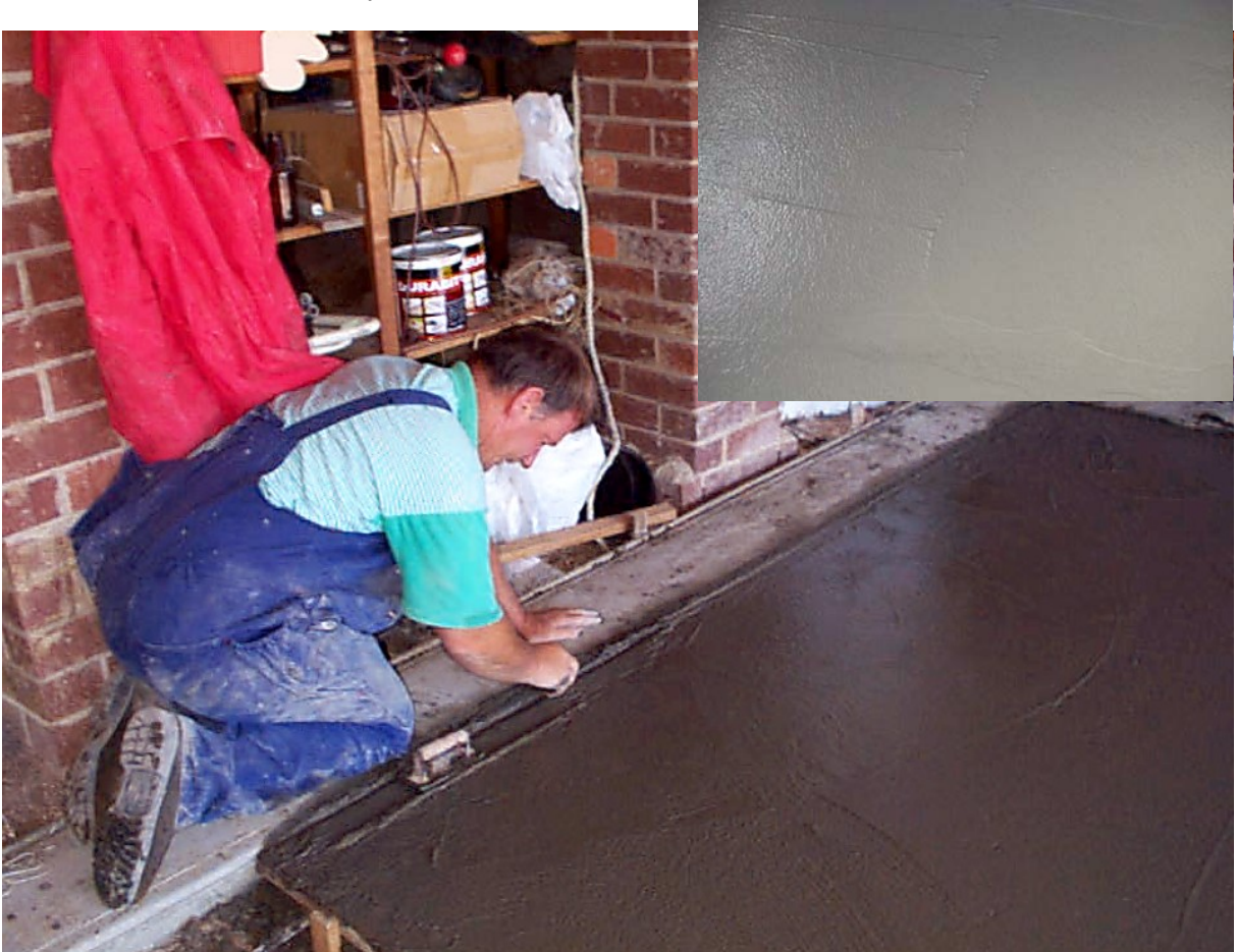
Figure 2 - Mike Burdon Finishing Off the Edges of a Low Slump Placed concrete with an Edging Tool. Insert – The Silky Finish Obtained
